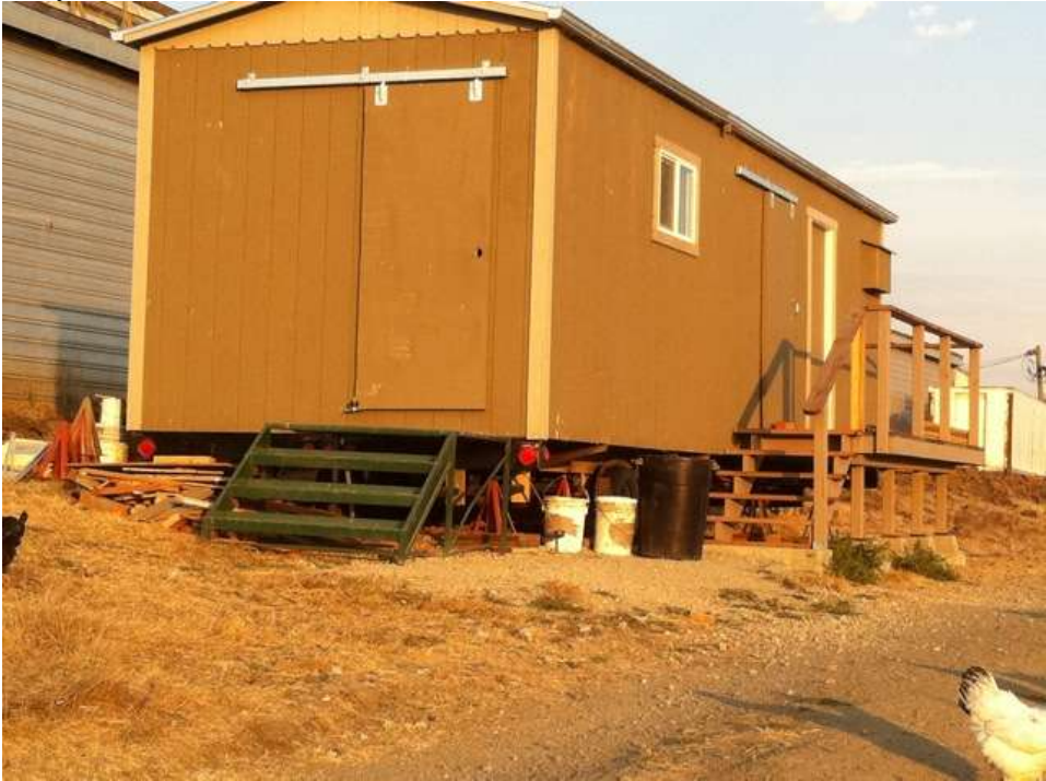
Dairy Exterior (under construction)
