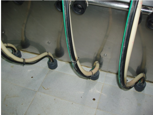
Milk hoses going to lower level
